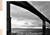
Figure 3: A photograph of a large, modern bridge structure over water, likely the practice site.
